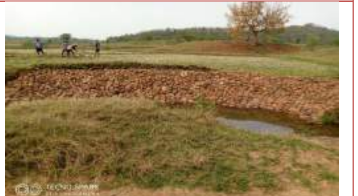
Stone patching (12mtr): Protect the field
